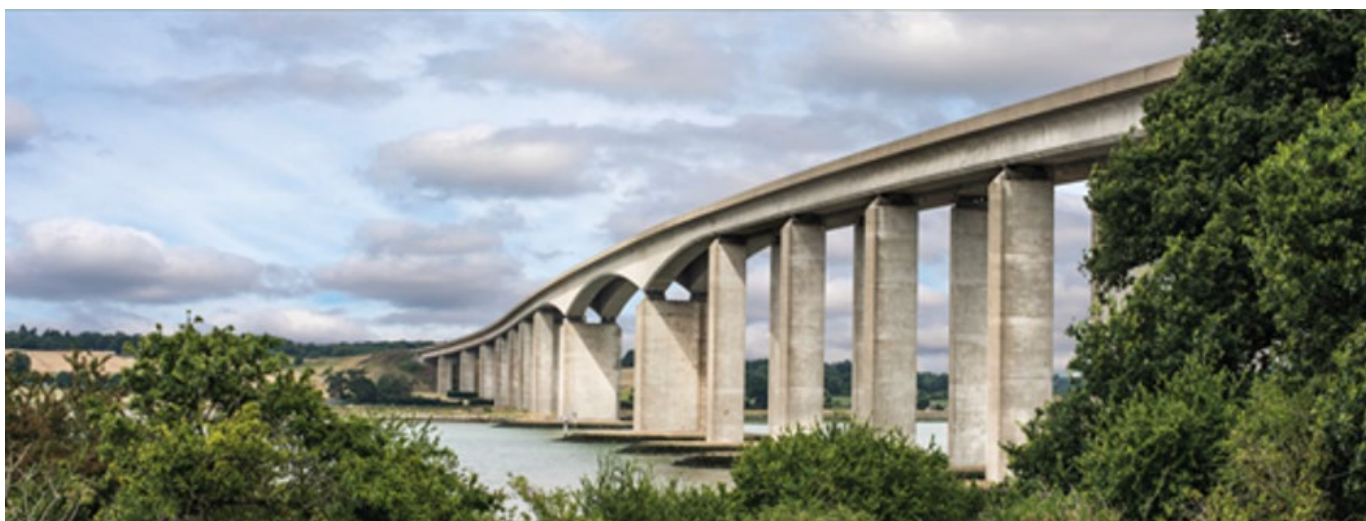
Orwell Bridge, Ipswich
